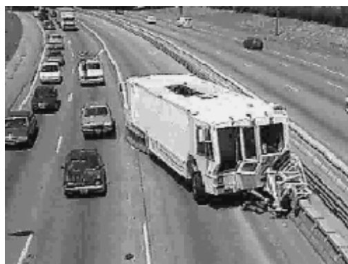
Fig. 4. Moving the concrete jersey barriers dividing the highway [17]
